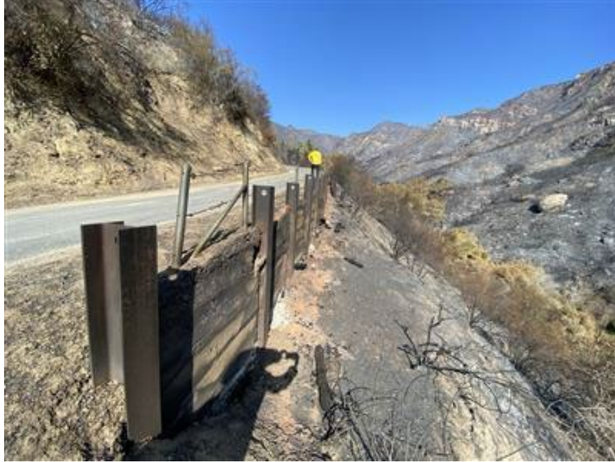
Fig. 2.53. Image of soldier pile wall with damaged timber lagging that retains soil along outside edge of road prism (34.059966°, -118.637916°).
