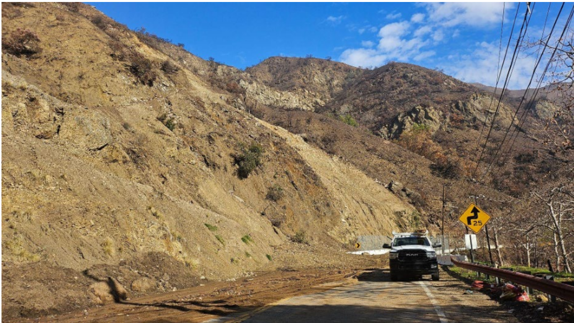
Fig. 2.18. Fine-grained sediments and rock debris from flood/flows accumulated near post mile 1.8 on State Route 27, where a landslide occurred in 2024. Metal mesh walls were damaged, and large boulders were transported downslope from steep terrain, with some remaining unstably positioned on the slope (coordinates: 34.063016°, -118.585803°).
