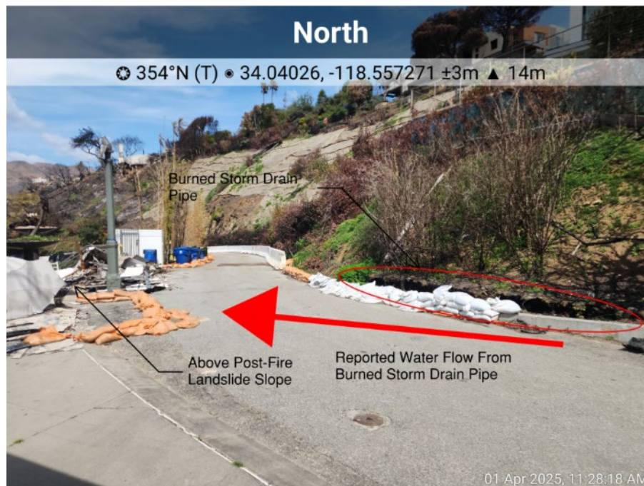
Fig. 2.26. Burned storm drainpipe in relation to the 2025 Castellammare landslide (4/1/25).
