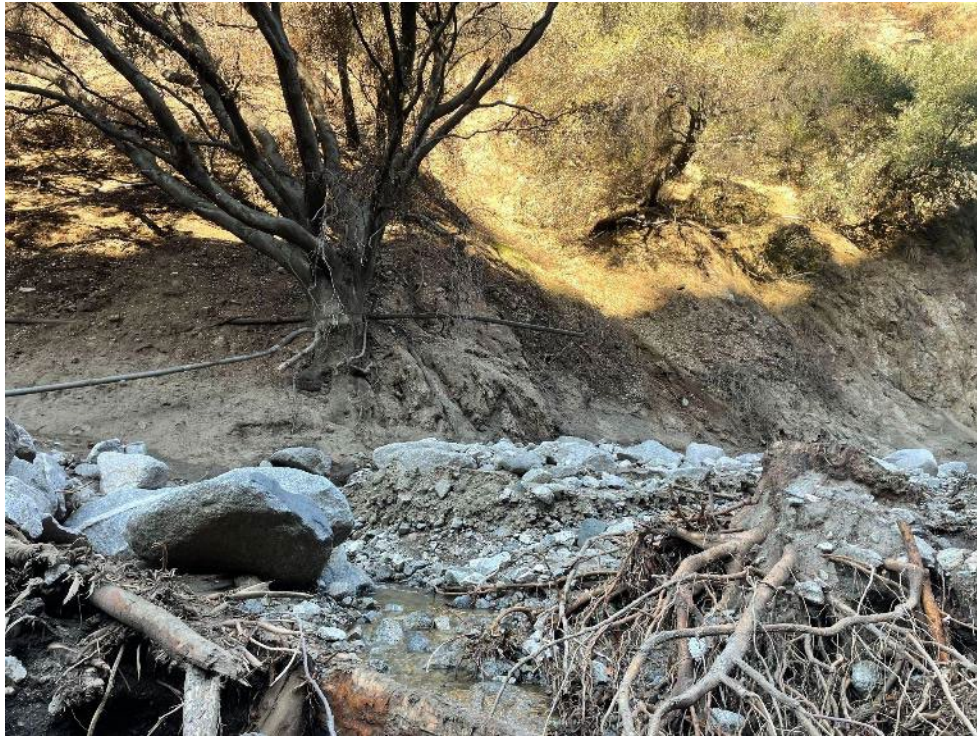
Fig. 3.17. Image showing damaged Kinneloa Irrigation District waterline (opposite bank) within Pasadena Canyon. Several waterlines of different ages exist along this reach. Observed damage occurred during the February 13th, 2025, storm. Photo taken on 2-20-2025. (34.18294°, 118.07856°).
