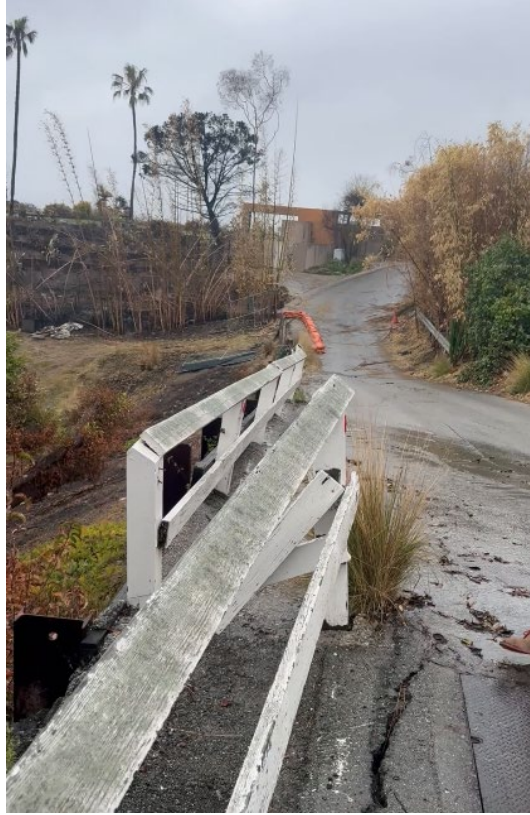
Fig. 2.27. Storm water diverted to descending slope due to burned storm drainpipe (photograph from video courtesy of Elaine Culotti) (coordinates 34.04041667°, -118.5567167°).
