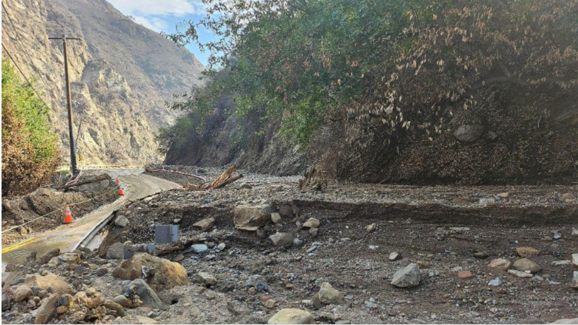
Fig. 2.17. Debris flood deposits near State Route 27 in Topanga Canyon. Damaged roadside rails resulted from flow impacts. The exposed deposit wall reveals stratification in flow near the surface (coordinates: 34.070734°, -118.588038°).
