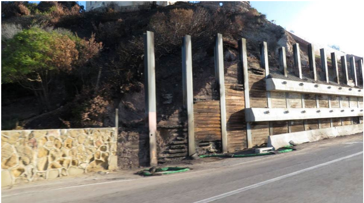
Fig. 2.52. Soldier pile with timber lagging retaining wall with tie-backs along Pacific Coast Highway. The timber lagging was burned in some locations (2/4/25).
