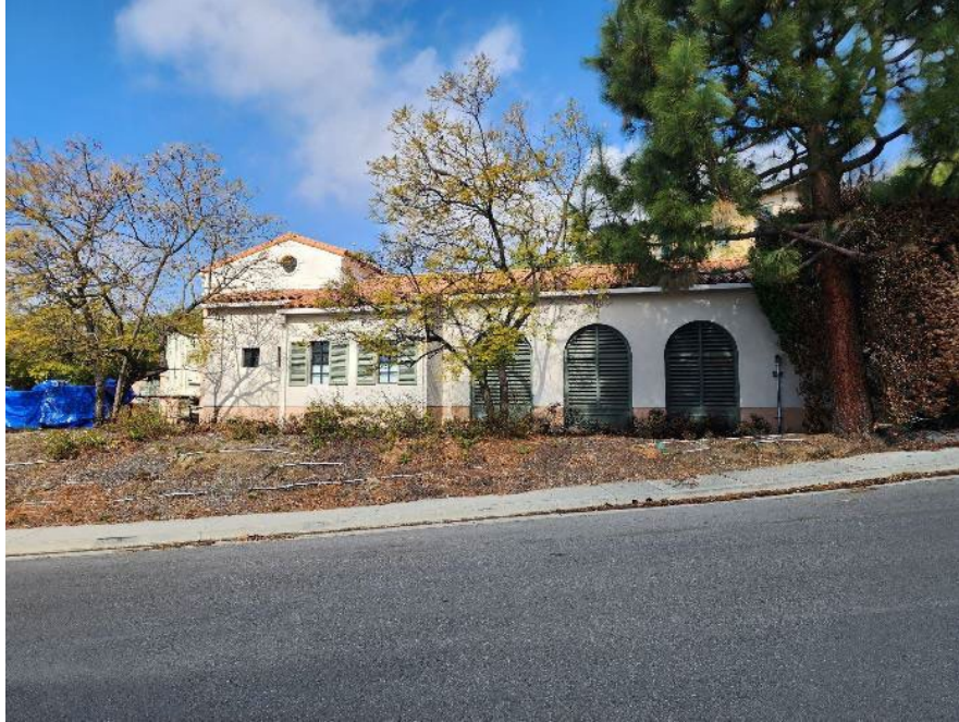
Fig. 2.37. Photograph of the LADWP Trailer Pump Station in Palisades Highlands (architecturally disguised to appear similar to residential structures) in the burn area. Many burned houses were in the vicinity of the pump station (34.07438131°, -118.550311°).
