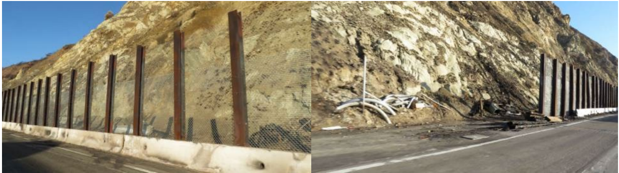
Fig. 2.59. Soldier pile and wood lagging rock barrier wall along the Pacific Coast Highway in Malibu area. The wood lagging completely burned out and was replaced with chain link fencing soon after the fire. The photo on right shows remaining evidence of the burned out wood lagging (February 4, 2025).
