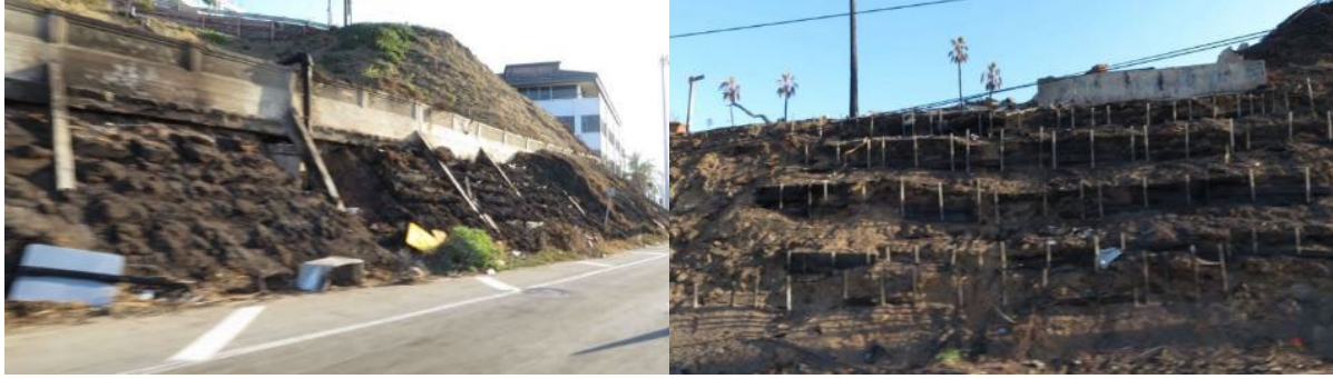
Fig. 2.55. Images of wood lagging completely burned out. The wood lagging supported slopes at several locations along the Pacific Coast Highway prior to the fire (2/4/25).
