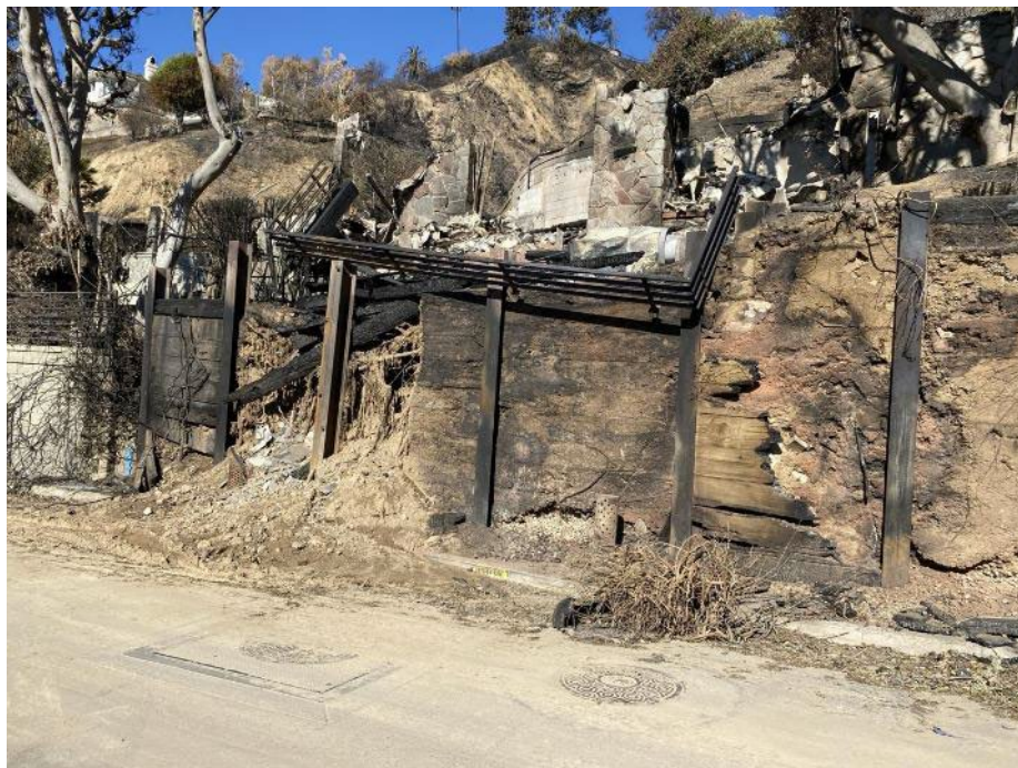
Fig. 2.54. Image of soldier pile wall with damaged timber lagging that retains soil along outside edge of building pad that supports foundation of a burned structure (34.0408°, -118.64546°).
