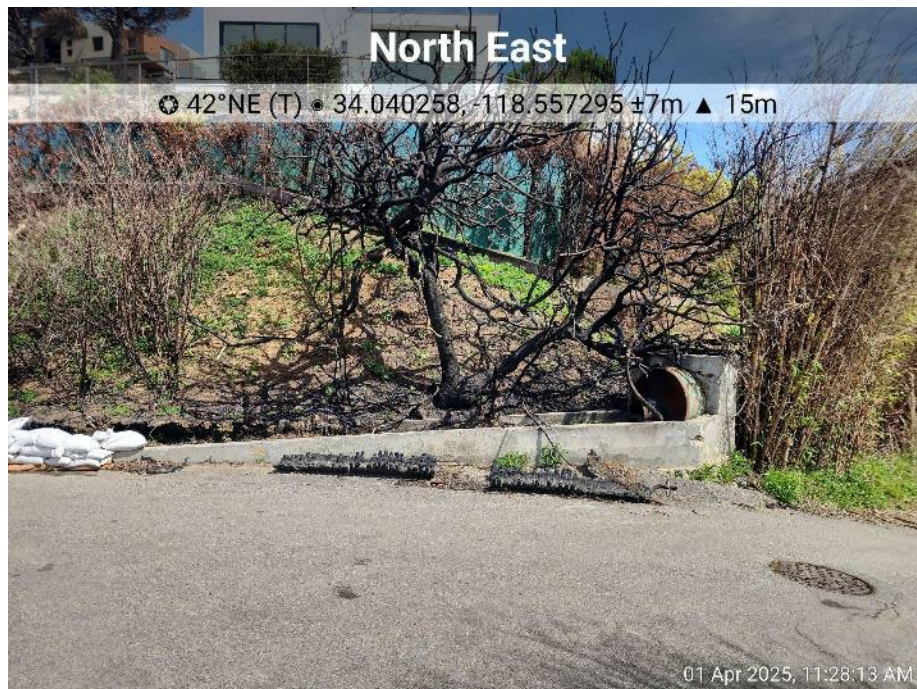
Fig. 2.25. Storm drainpipe completely burned on Revello Dr., upslope of the 2025 Castellammare landslide (4/1/25).
