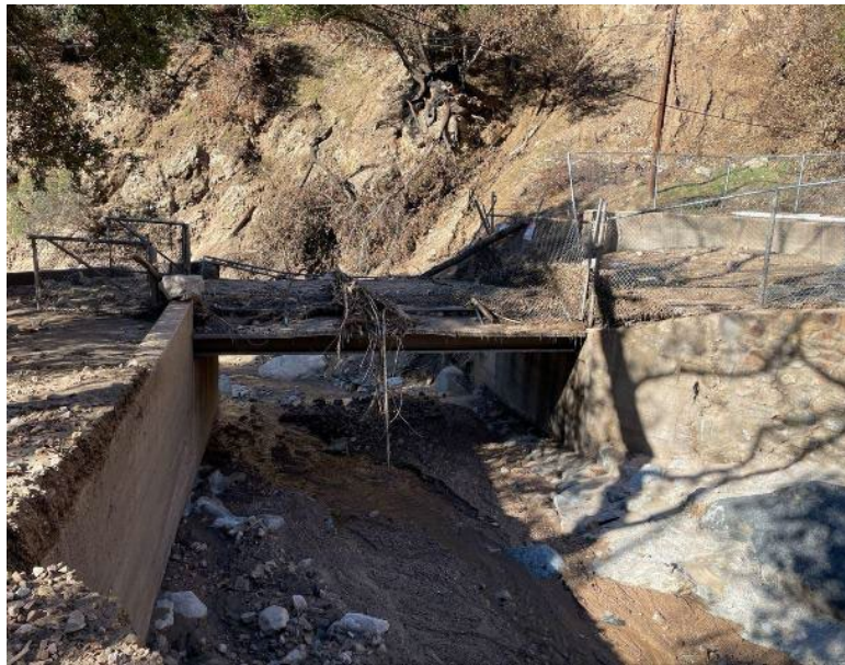
Fig. 3.16. Damage to the bridge and associated fencing (2/19/25, 34.18385°, 118.12288°).
