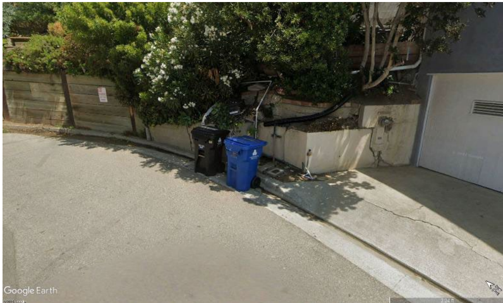
Fig. 2.28. Google Earth image from 8/22, showing a failing retaining wall at rear of the house with several drainpipes draped over the wall.
