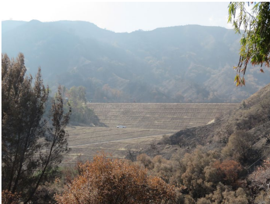
Fig. 2.38. Photograph of the LADWP Santa Ynez Reservoir Dam in Palisades Highlands in the burn area showing straw wattle to protect against future erosion of the compacted earth embankment after the fire burned the natural ground cover (34.073142°, -118.569466°).
