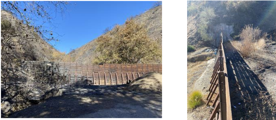
Fig. 2.34. Photograph of a partially burned debris retention structure (34.1061, -118.50564) in Mandeville Canyon before the January storm.
