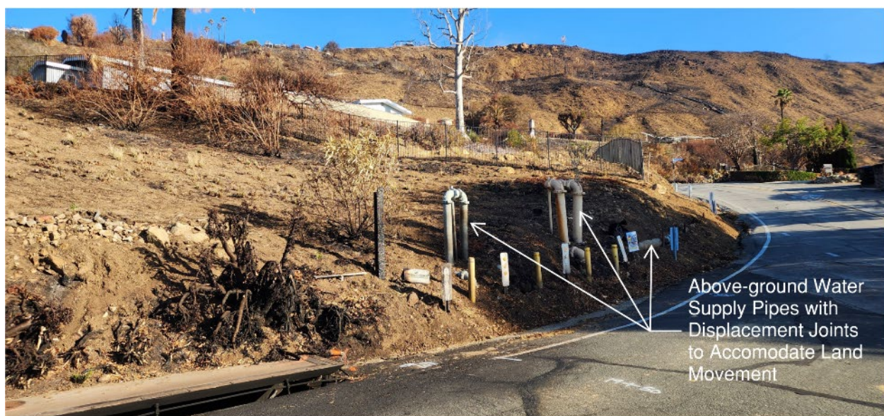
Fig. 2.35. Photograph of above-ground water supply pipeline with slope-movement mitigation expansion joints (34.0412773°, -118.6194627°) in Big Rock Mesa area.
