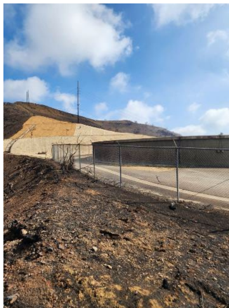
Fig. 2.36. Photographs of the Temescal Tank circular water supply tank in Palisades Highland. Recent slope erosion mitigation (with jute mesh) had been performed behind the tank (likely post-fire), and some of the ancillary equipment attached to the tank may have been recently repaired based on observations, some equipment was scorched by the fire. (34.0777306°, -118.546853°).
