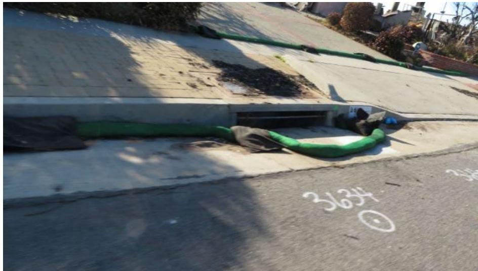
Fig. 2.41. Surface runoff and storm drain basins protected against spread of contaminants (2/4/25).
