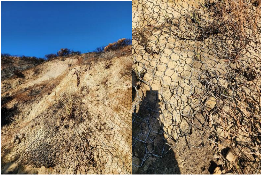
Fig. 2.50. Rock netting with discoloration indicating fire exposure in Palisades Fire. Big Rock Dr., Malibu (2/4/25).
