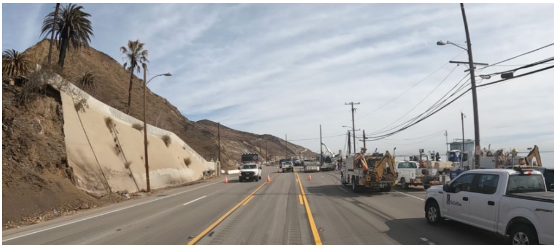
Fig. 2.58. Shotcrete-treated slopes along the Pacific Coast Highway remained largely undamaged.
