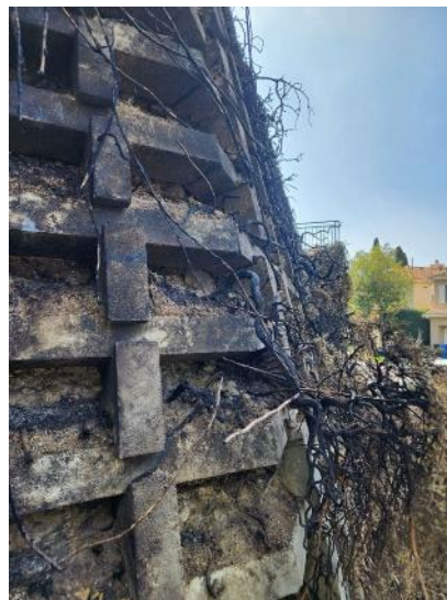
Fig. 2.56. Crib Wall with Burned Surficial Vegetation and Fire Exposure in Palisades Fire. (a) Post-Fire, (b) Pre-Fire Google Street View Image, (c) Close-Up of Burned Surface. Calle Patricia at Calle Jermaine, Palisades Highlands, Pacific Palisades (a and c taken 2/4/25).
