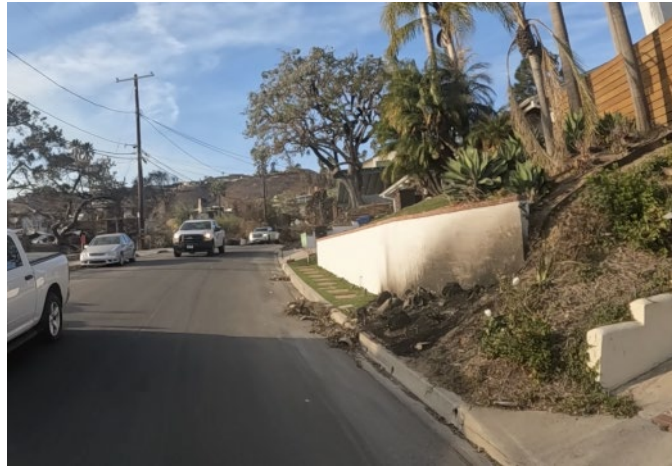
Fig. 2.57. Stucco-faced short retaining wall remains intact, with debris accumulation above the slope.
