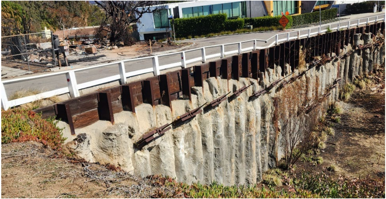
Fig. 2.51. Soldier beam and tie-back anchor retaining structure with combination of timber and shotcrete lagging. Upper edge of Tramanto Dr. Landslide, Tramanto Dr., Castellammare, Pacific Palisades (2/4/25).
